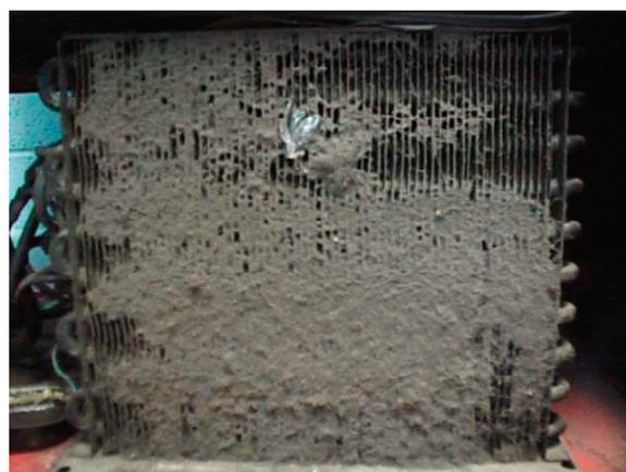
*A dirty condenser block can be the cause of high discharge pressures.*
