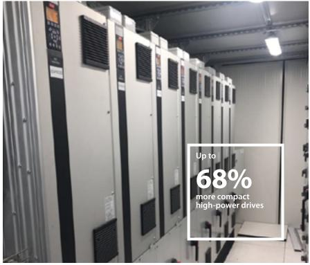
The extremely powerful and compact VLT® AQUA Drive in enclosure size D regulates flow rate, and is a fundamentál component in minimizing energy consumption.
