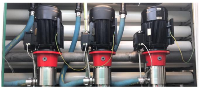
**Mr Tota explains:** "iSave devices, which recover the hydraulic energy of the reverse osmosis process discharge flow, drastically reducing energy consumption, are extremely compact and can be integrated with Danfoss high-pressure pumps"
