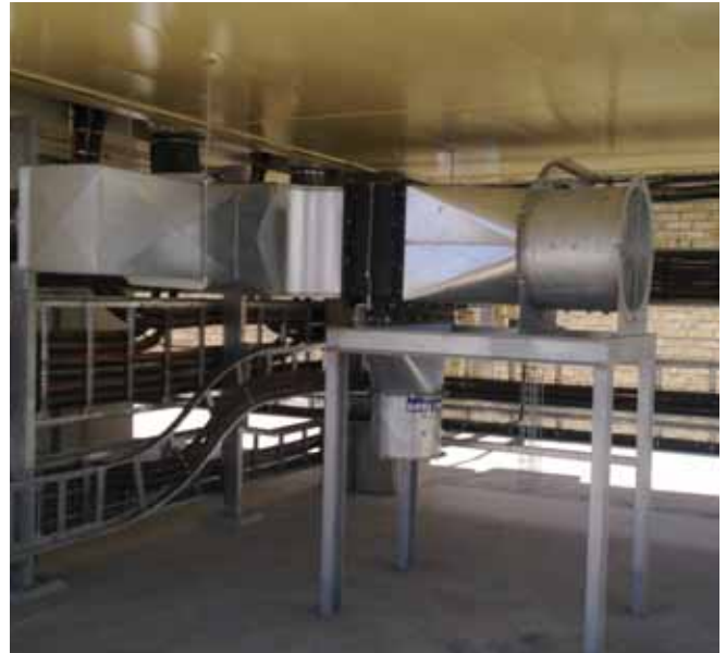
Maintenance-free spin filter system removes dust from air before it enters the heat sink channel of the frequency converter.
