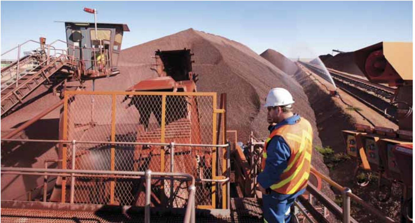
A stacker-reclaimer in action at Kolomela
