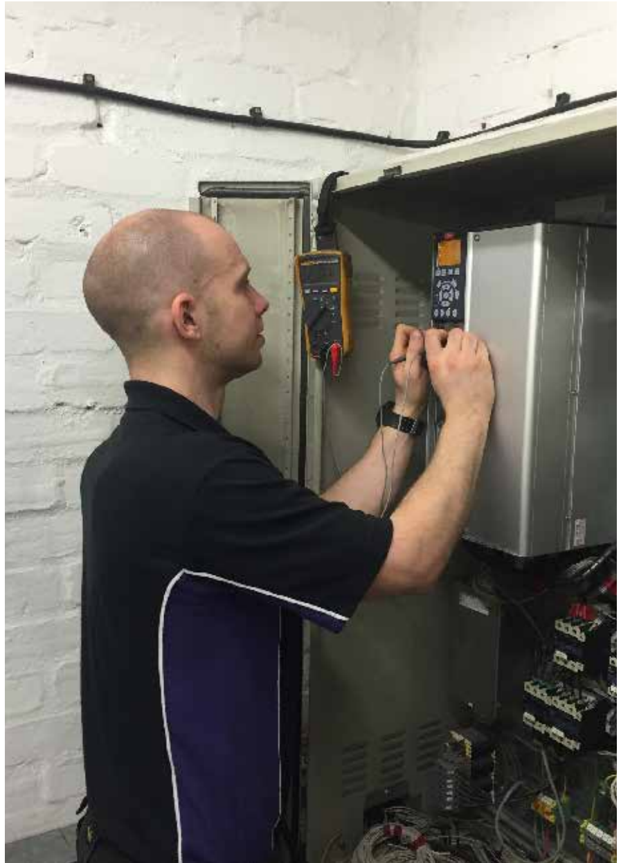
Ben Fordham of Northern Industrial fitting the drive on site
