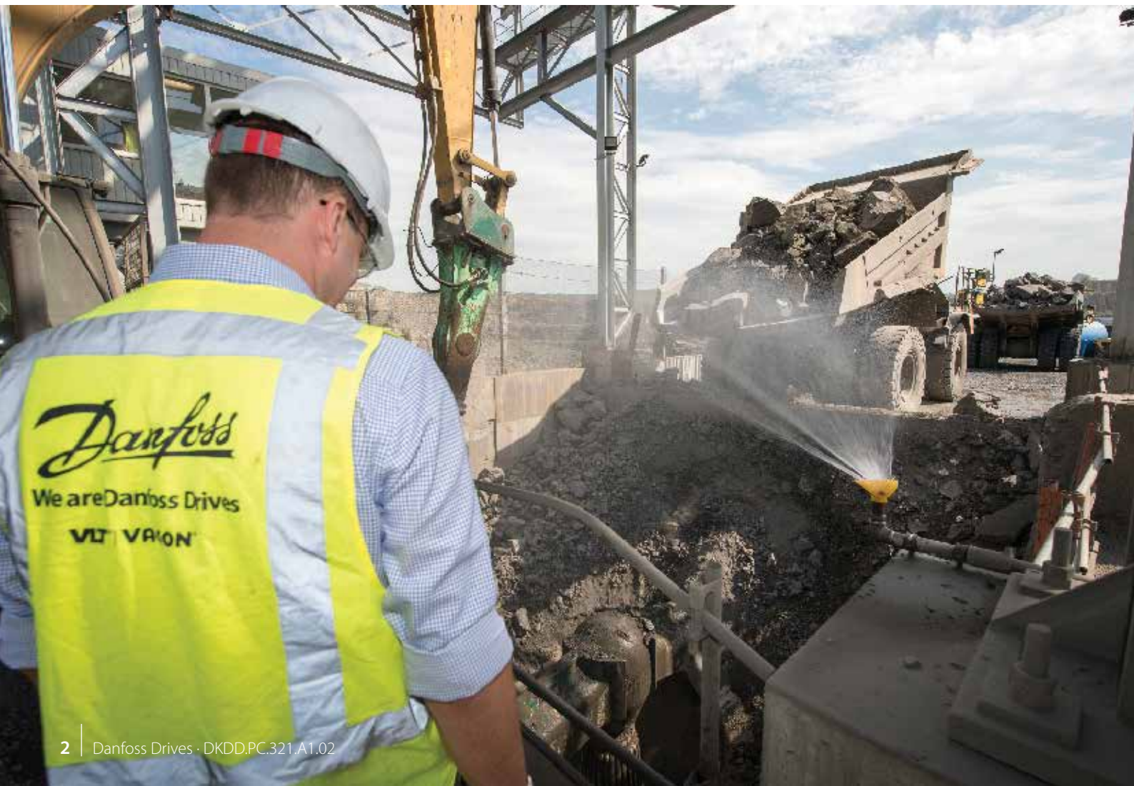
Unloading quarried limestone into the crusher.
