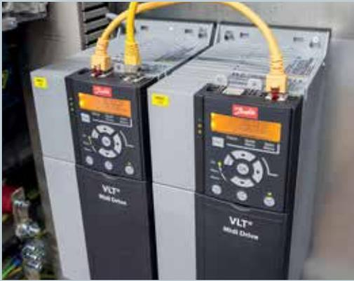
*Tresch Automation chose the Danfoss VLT® Midi Drive FC 280 to control the speed of rotation which is defined by the system. The winemaker can then adjust the speed up or down by a few percent using a keypad.*
