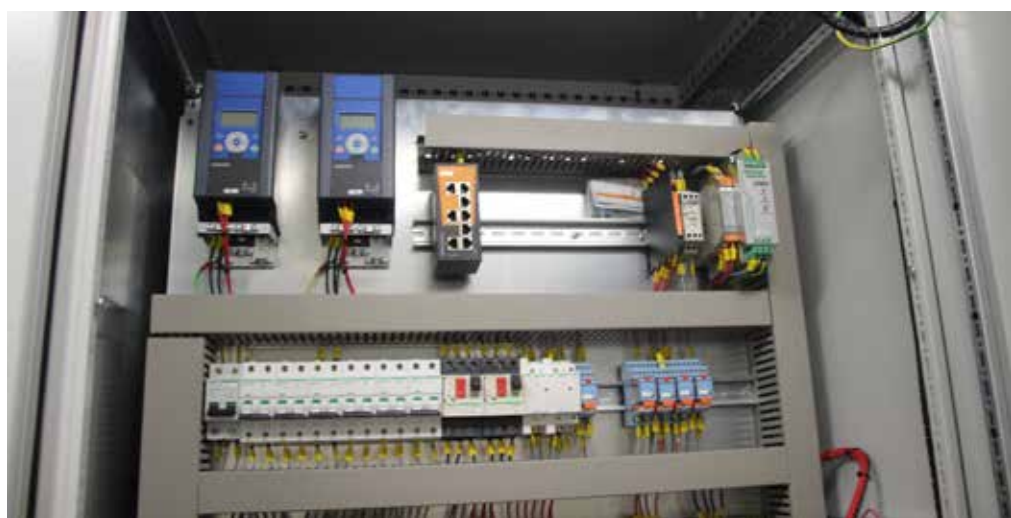
Wiring field with good access. Also the ventilation fans for the container are powered by VACON® drives.
