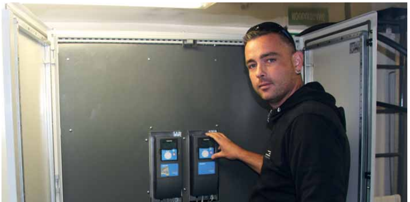
Dominic van der Meer with the VACON® Liquid Cooled Drives
