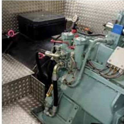
Main diesel engine with shaft motor
