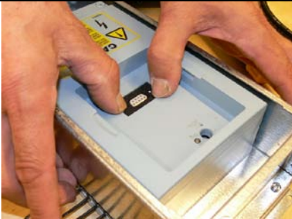
13. Attach the seal around the RS485 connector.
