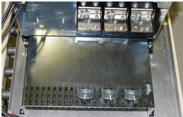
Figure 11. Cable-clamp bracket mounted on E2 frame.
