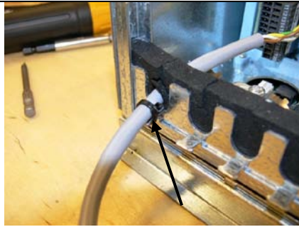
11. Attach the cable to the washer with a plastic binder
