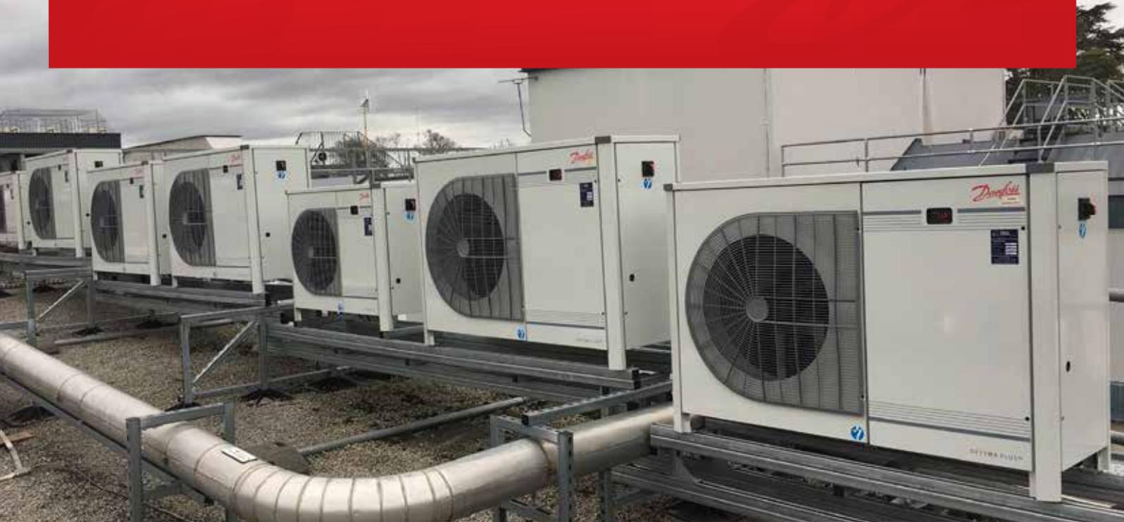
**When a busy hospital needed to relocate its cold room condensing units, Consultant Neil Garnett knew it was time to upgrade to F-Gas compliant refrigerants. He chose Optyma™ Plus units, running with R134a and – crucially – R452A.**
