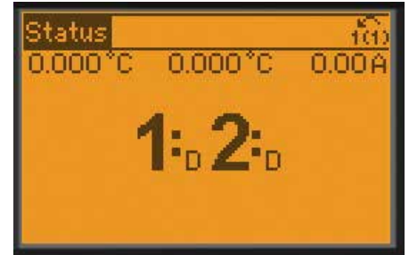
The compressor status can be read directly from the display.
