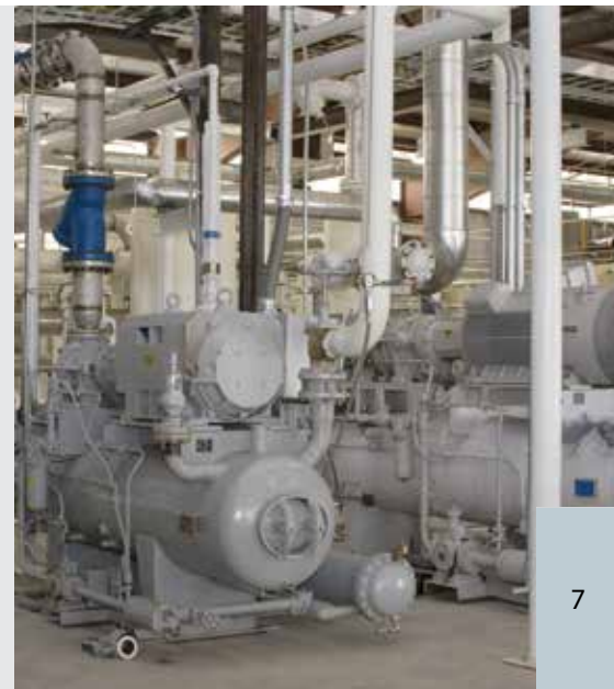
Speed Control of lead Compressor plus one more, offers improved and streamlined design possibilities and a better choice of Compressors sizing to adapt to varying load conditions
