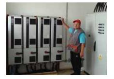
moisture. All the frequency converters have an integrated mains disconnect and fuses.
