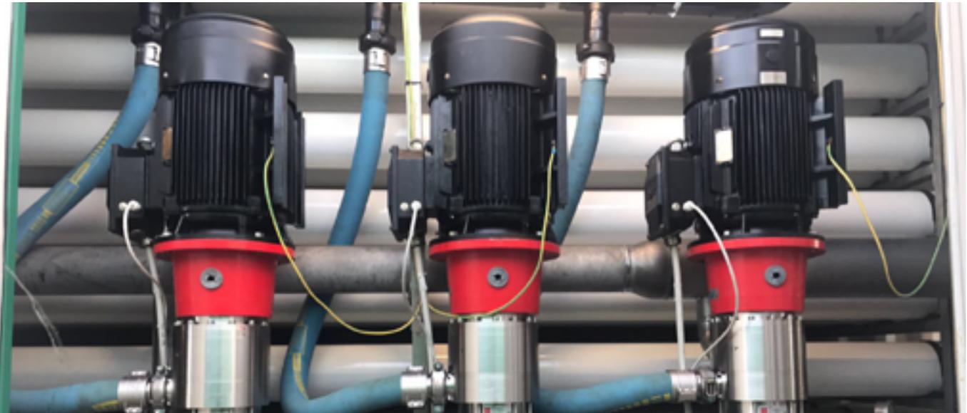
**Mr Tota explains:** “iSave devices, which recover the hydraulic energy of the reverse osmosis process discharge flow, drastically reducing energy consumption, are extremely compact and can be integrated with Danfoss high-pressure pumps”
