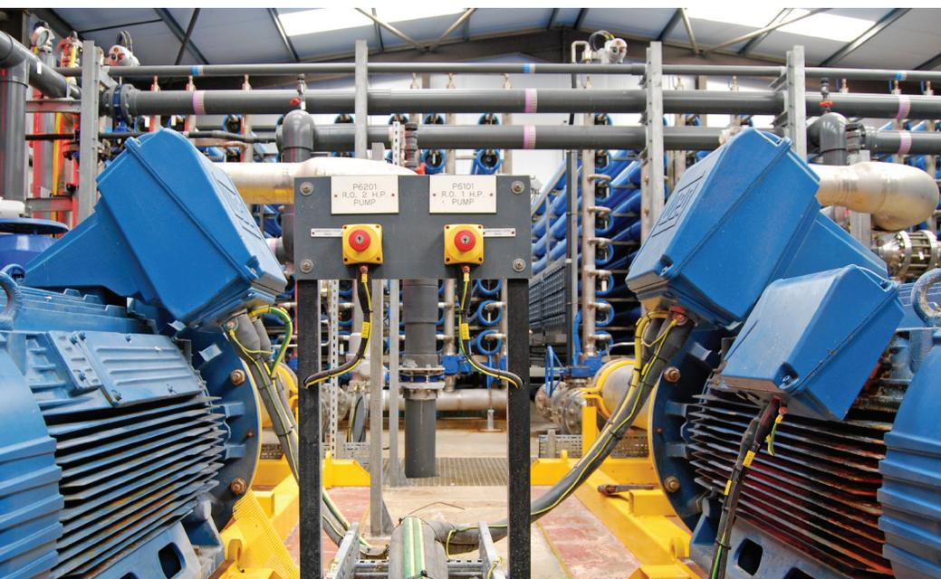
The upgrade involved the installation of a large number of new pumps, almost all of which would need to be controlled by AC drives.
