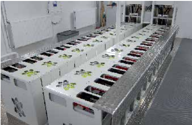
The 2 x 65 kWh Li-Ion EST-Floatch Battery system with battery management system.
