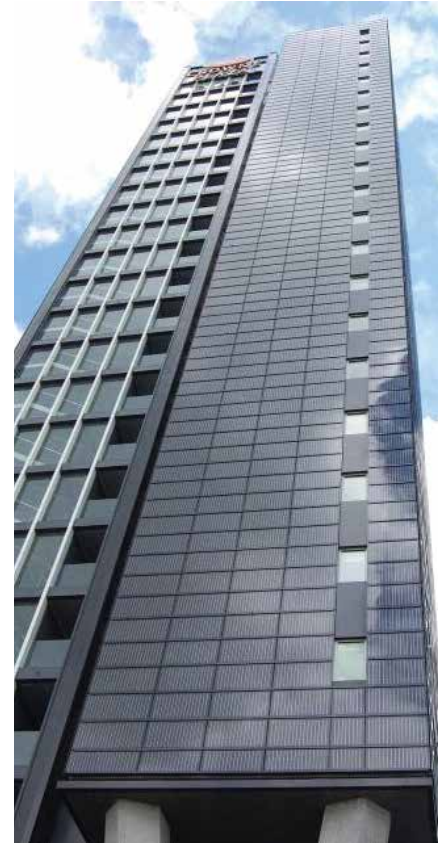
2,500 m 2 specially adapted solar cell panels are mounted on three of the hotel's four facades. They generate 10% of the electricity consumption of the hotel.
