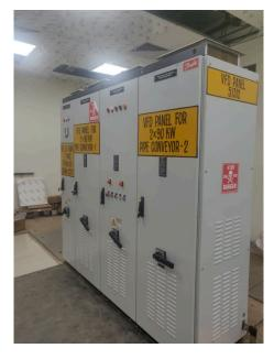
motor itself as well as on any load present in the equipment. With a VFD, the amount of torque applied is accurately controlled, permitting equipment start-up at zero velocity with a smooth acceleration up to normal operating speed. In addition, with a VFD, a motor torque limitation threshold is set which prevents equipment damage in the event of a jam or other catastrophic event.
