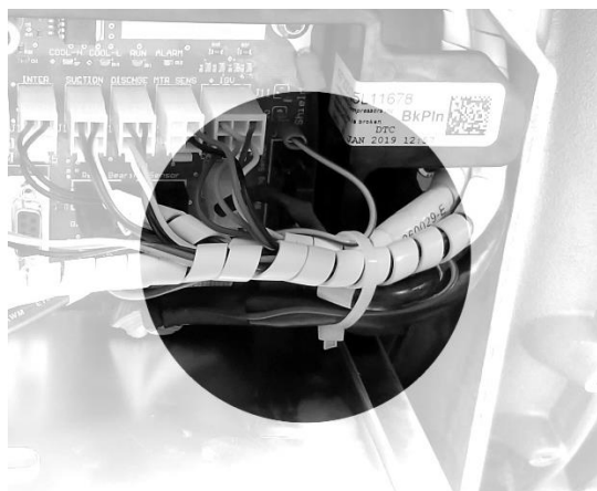
Figure 15 – Backplane Harness Cable Tie
