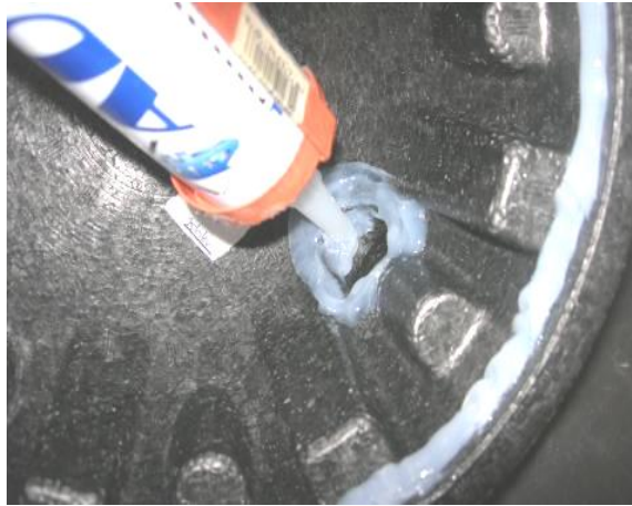
Figure 3 Silicone Sealant Inside Eyebolt
