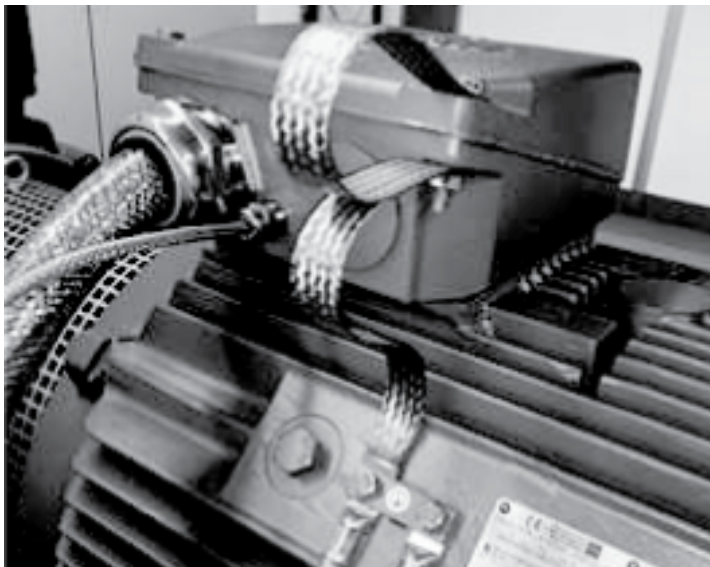
Illustration 2: Installation of EMC straps from the Terminal Box to the Motor Frame
