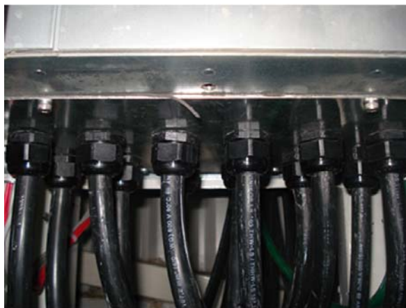
Figure 3.25: Example of proper installation of the gland plate.
