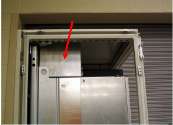
Photo 8. Top duct work and enclosure top installed.
