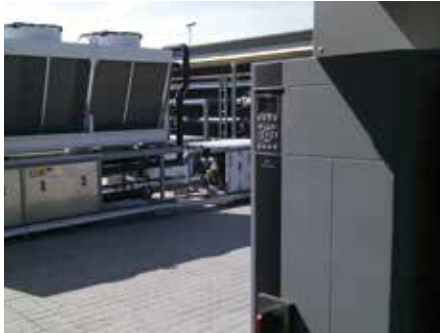
The VLT® HVAC Drive withstands outdoor environments. A NEMA/UL Type 3R rated enclosure, and standard 1,000-foot motor cable runs, provide maximum mounting flexibility.
