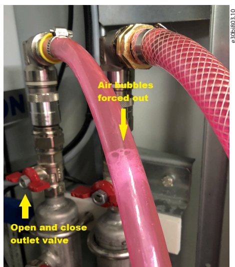
Illustration 75: Removing the Air
