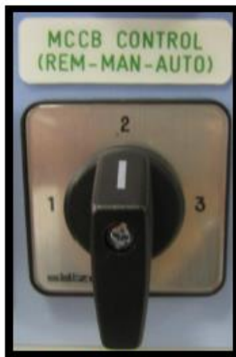
Figure 7-1. MCCB Control selector switch (-S6)
