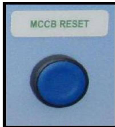
Figure 7-6. MCCB Reset push-button (-S11)
