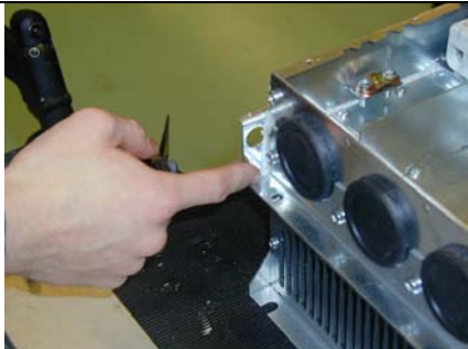
10. Smoothen all sealed seams with your finger. Tip your finger in soap water before smoothening the seams.
