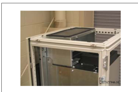
Illustration 3.46: Øvre kabel installeret
