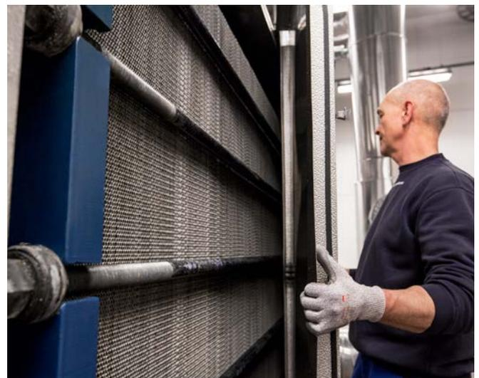
*Replacing the old heat exchangers' plates with new ones at AffaldVarme Aarhus*
