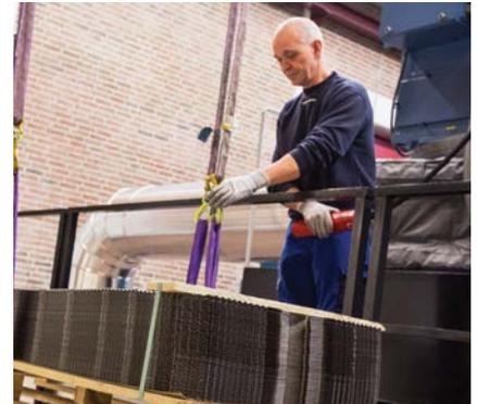
Replacing the old heat exchangers' plates with new ones at AffaldVarme Aarhus
