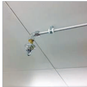
SEM-SAFE® high-pressure water mist nozzle from Danfoss.
