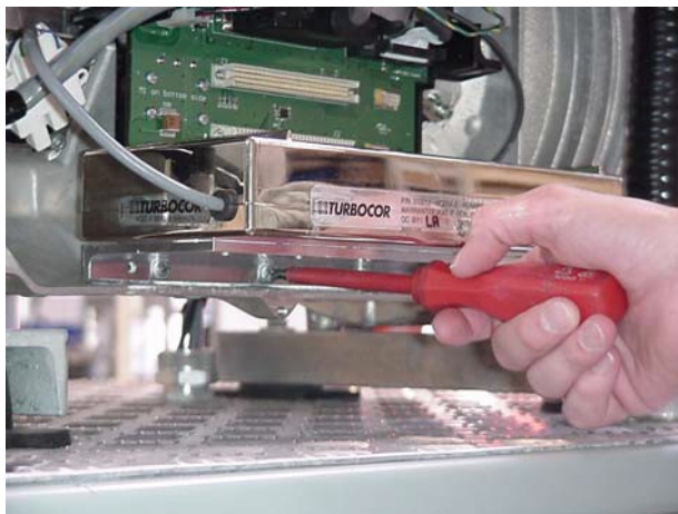
Figure 2 - Removing the PWM Amplifier
