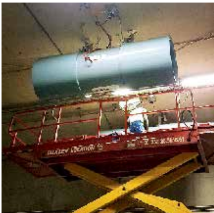
Working on a ventilation unit.
