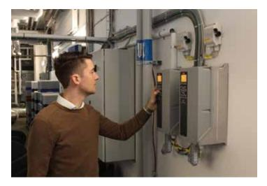
Jacob Haulrich, Nordomatic, continues: "We also use the new VLT® Pressure Transmitter PTU 025 pressure transmitter unit, which monitors air filter clogging and air volume through the ventilation fans. We can obtain the values via BACnet, and because this unit has four pressure transmitters, it has resulted in elimination of three pressure sensors, including cabling, per system".
