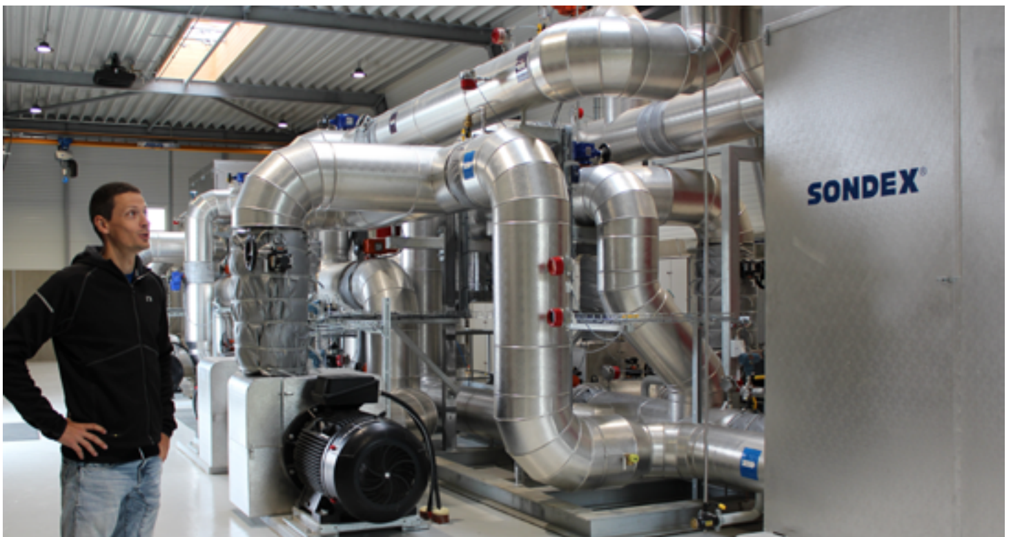
During a guided tour, Per Hvilshøj Christiansen gave an introduction to the heat transfer solution by SONDEX®.
