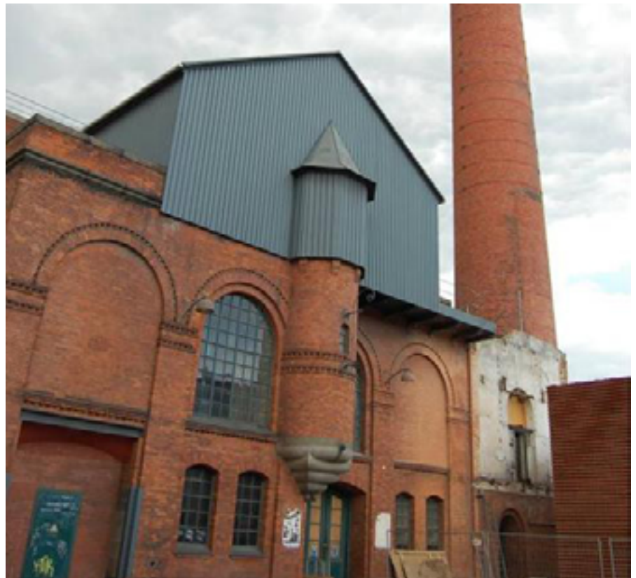
A former power plant near the Kongens Nytorv square in central Copenhagen has been given a new lease on life. From here, Denmark's first large-scale district cooling plant supplies large commercial buildings such as banks, hotels, office buildings and many other companies, with cost-effective, environmentally friendly cooling.
