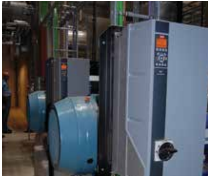
IE4 SynRM motors equipped with VLT® AutomationDrive FC302 frequency converters.
