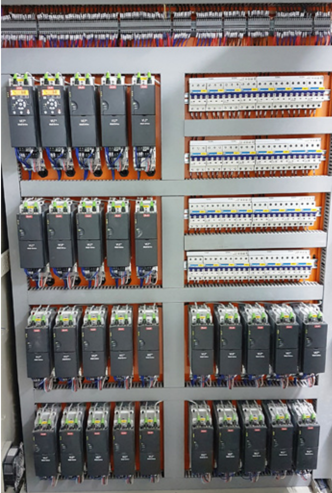
VLT® Midi Drive FC 280 and VLT® AutomationDrive FC 302 with Integrated Motion Controller installed side-by-side.
