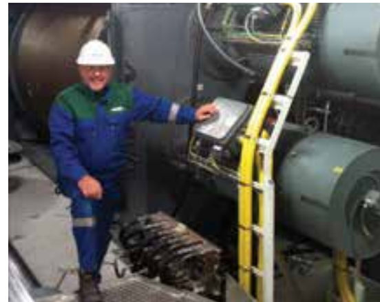
Active heave compensation (AHC) systems are increasingly being deployed to complement deep water installation applications. Active heave compensated winches are designed to enable equipment to be safely lowered to and lifted from the sea bed during high seas. Advanced fiber and carbon ropes are being used instead of heavy steel cables.
