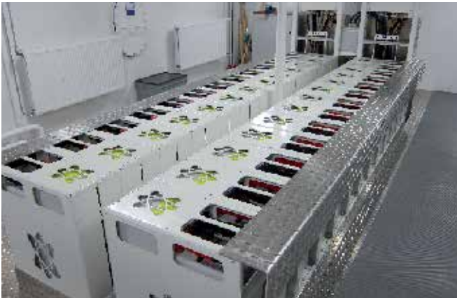
The 2 x 68 kWh Li-Ion EST-Floatch Battery system with battery management system.
