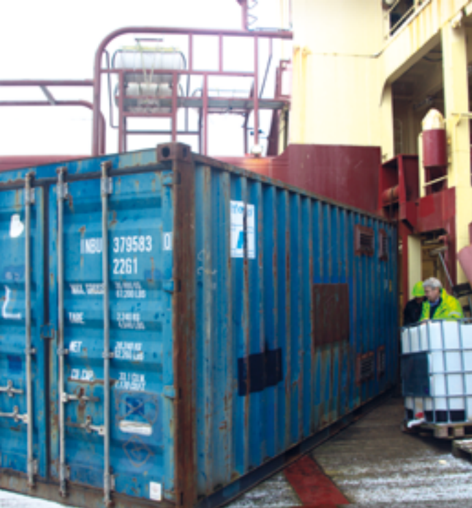
The VLT® drives are cooled with the back channel cooling system which draws cooling air in and out directly via the vents in the container wall.
