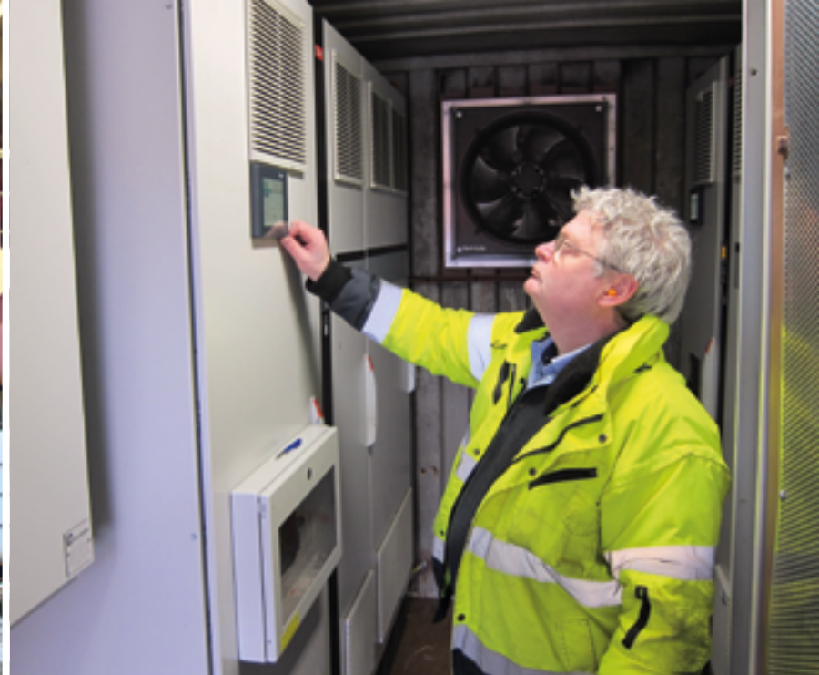
The VLT® drives are cooled with the back channel cooling system which draws cooling air in and out directly via the vents in the container wall.
