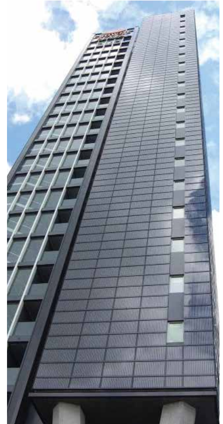
2,500 m 2 specially adapted solar cell panels are mounted on three of the hotel's four facades. They generate 10% of the electricity consumption of the hotel.
