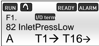
Figure 7.1-4, Low pressure alarm on the NXP panel
