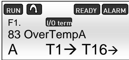
Figure 7.1-2, High temperature alarm on the NXP panel
