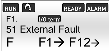
Figure 7.1-5, Leak alarm on the NXP panel
