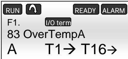
Figure 7.1-2, High temperature alarm on the NXP panel
