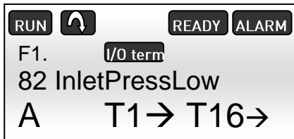
Figure 7.1-4, Low pressure alarm on the NXP panel
