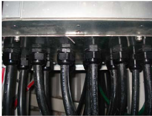
Illustration 4.16: Example of proper installation of the gland plate.
