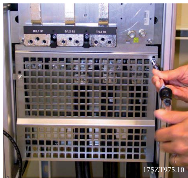
Illustration 3.12 Mounting of EMC shield.
